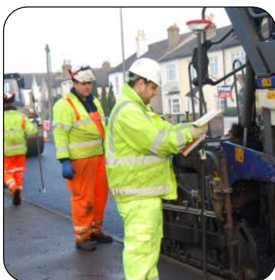
Figure 5 – Material extents per truck recorded using GPS
